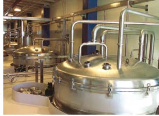
Multi-distribution system on top of calandria
