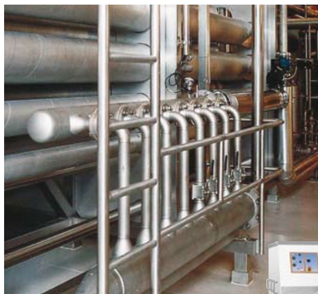
Tangential swirl heater for direct steam injection
