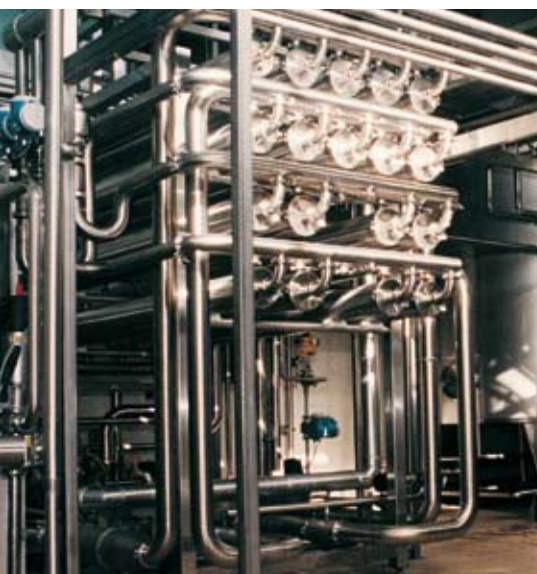
Ultrafiltration plant for whey
